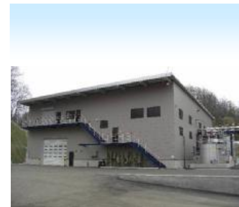
Plant for impure residues
