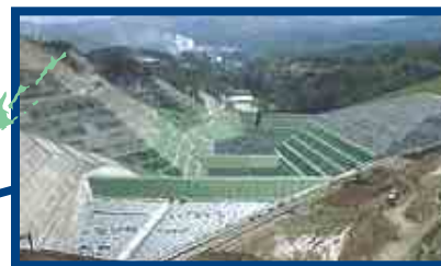
The largest private-sector managed final disposal facility (Kosaka, Akita Prefecture)
